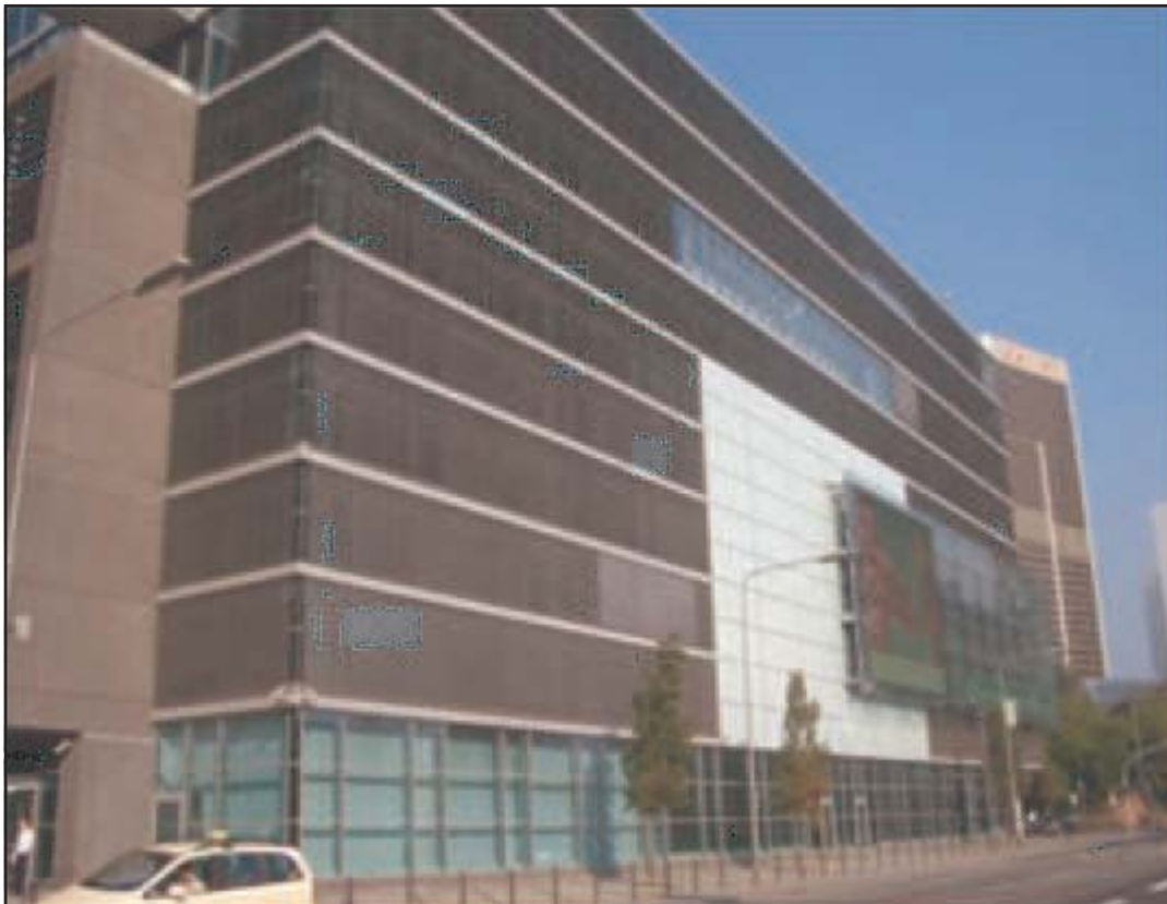
One of the Frankfurt office properties used by Dresner Bank to house its Dresner Kleinwort Wasserstein investment banking unit opposite the Frankfurt Exhibition Ground. It was contained in the €2bn portfolio of assets sold in December to the Eurocastle subsidiary of the US-based Fortress Investment Group .
