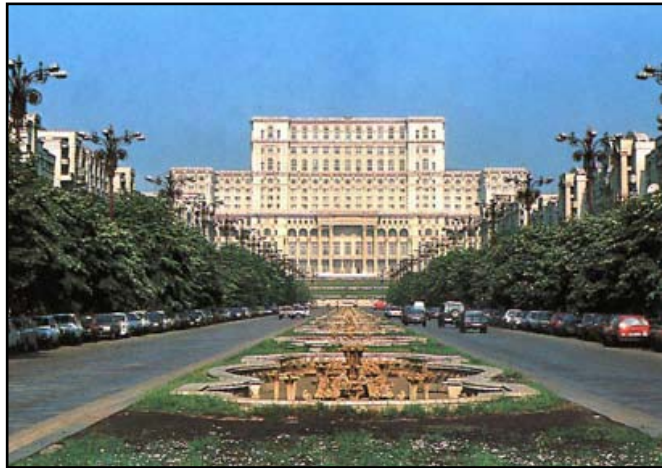
Bucharest's 3100-room House of the People built by Romanian dictator Nicolae Ceaucescu is the world's 2nd largest building after the Pentagon."
