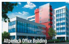
Altperlach Office Building
