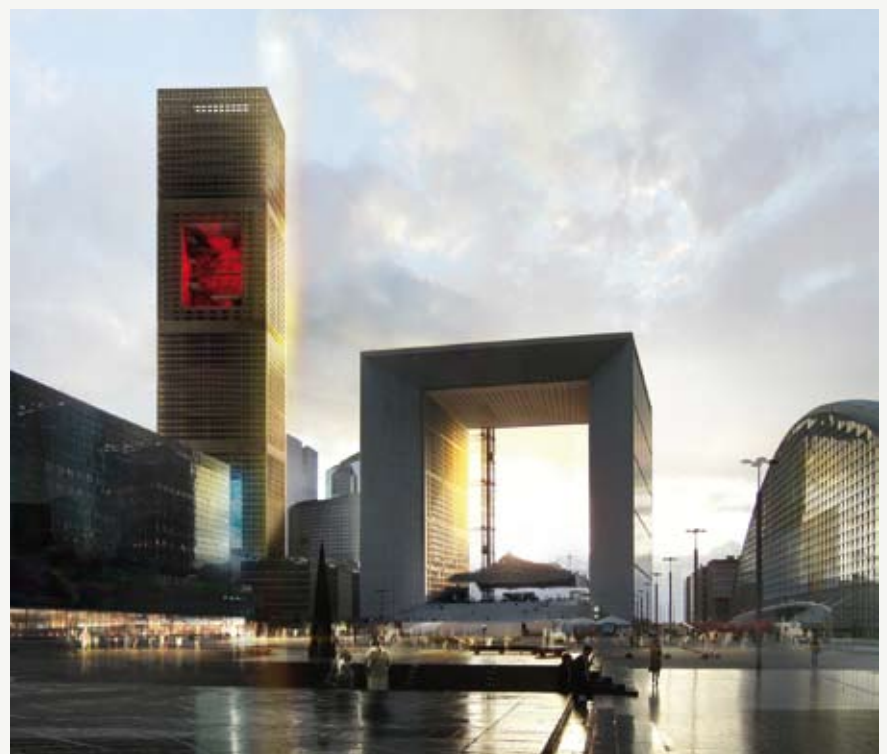
French architect Jean Nouvel's innovative design for the centrepiece Signal Tower of the new Paris La Défense (see here with the La Défense arch) is conceived as a structure 300m high, situated in the west, opening up the development toward Puteaux. It comprises 71 storeys in a mixed-use building, and is made up of four blocks, with atriums forming huge windows.
